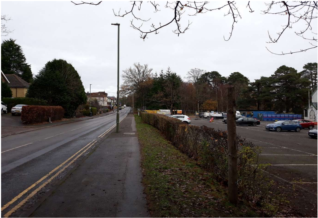
DEEPCUT BRIDGE ROAD LOOKING NORTH AND SOUTH (FORMER GARRISON CHURCH OF ST BARBARA AND ADJOINING MILITARY CEMETERY)
